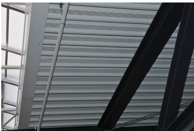
Departure hall with appr. 4.100 m 2 perforated trapeze sheet at the ceiling
